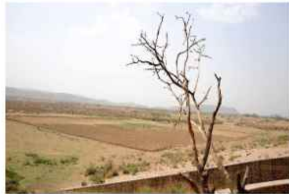
Under Performance of Water Resources Structures (Ramgarh Dam)
